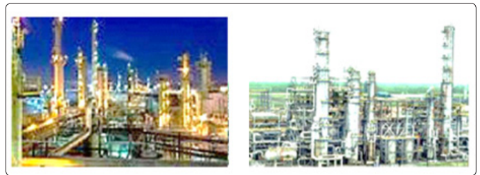
Figure 4a: Eleme Refinery
